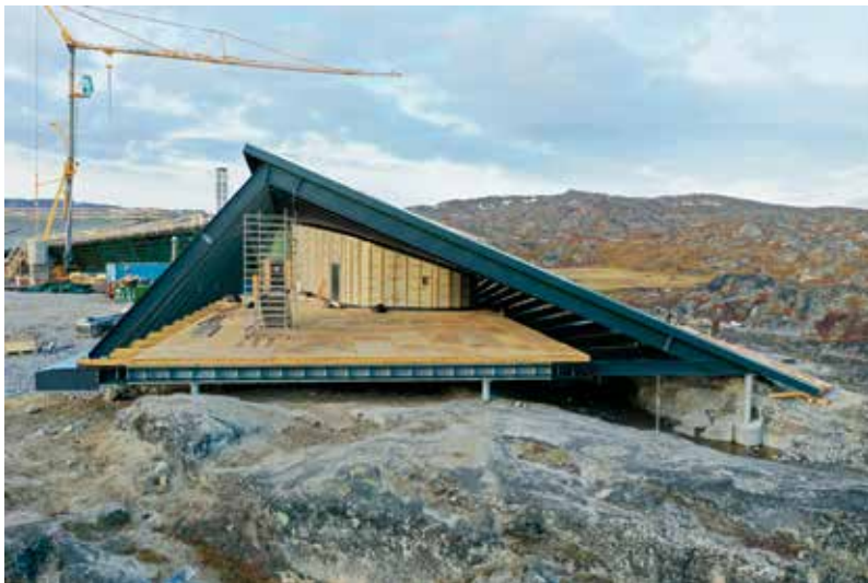
The Icefjord Centre under construction.
