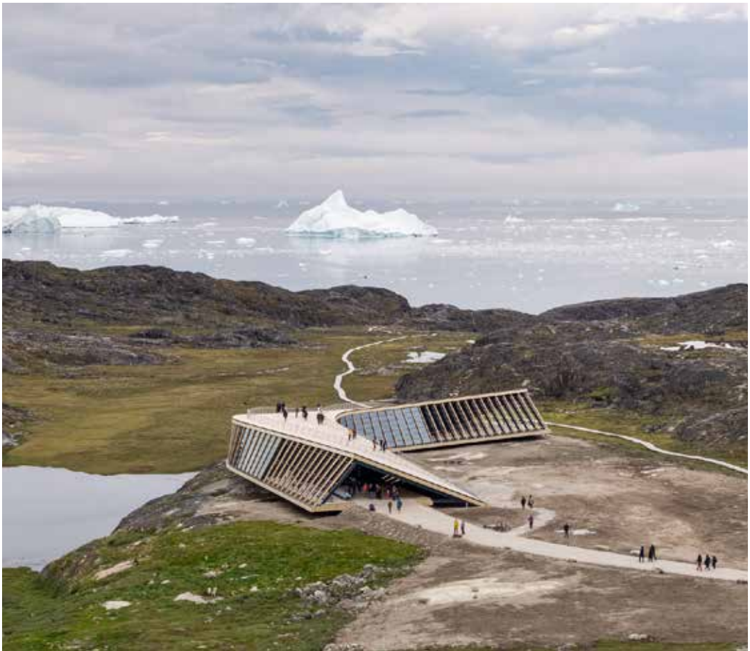
The Icefjord Centre has free access to the rooftop boardwalk, which offers stunning views of the mountains and the fjord.
